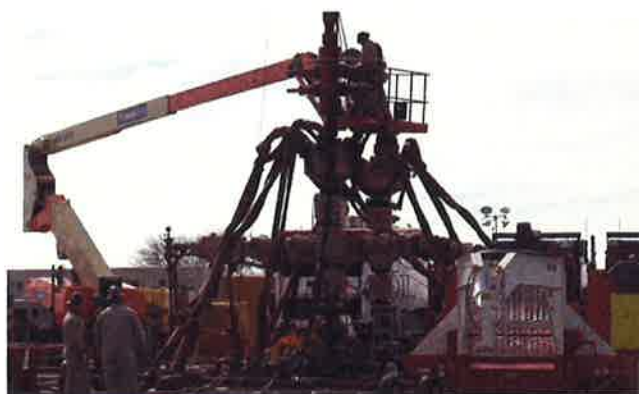
Figure 3. Traditional PCE Installation Involves Personnel Working At-Height With Heavy Hand Tools
